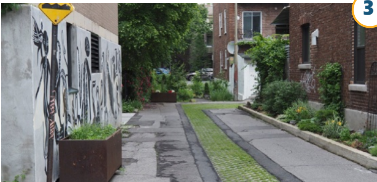
Figure 43. Example of a Permeable Alley Treatment
