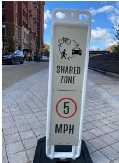
Figure 32. A Shared Zone sign in Chevy Chase, MD alerts drivers to expect and yield to pedestrians and other active transportation users.
