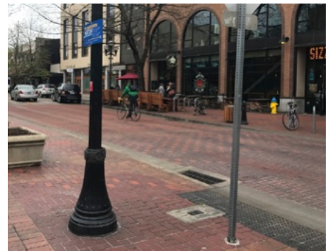
Figure 21. Example of Curbless Streets in Denver, CO; West Palm Beach, FL; and Eugene, OR, where the travel lane and zones are defined by planters, bollards, and other furniture elements.
