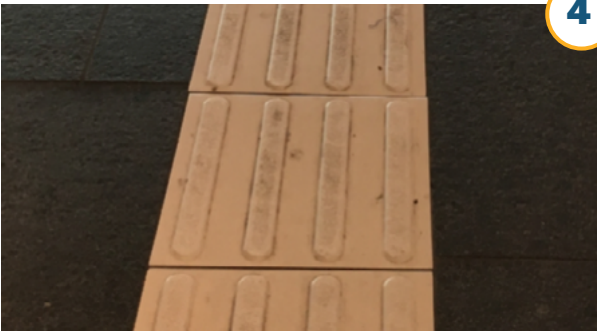
Figure 37. Example of tactile directional indicators
